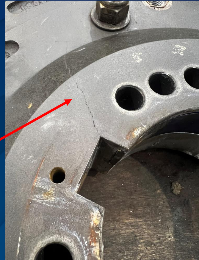
Crack in Logan clutch hub
