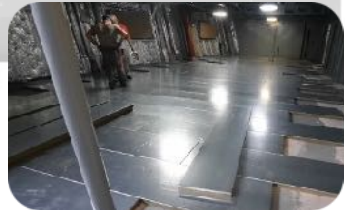
Labs insulation (walls & floor) with rock wool
