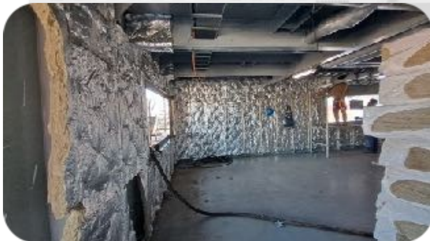
Labs insulation (walls & floor) with rock wool
